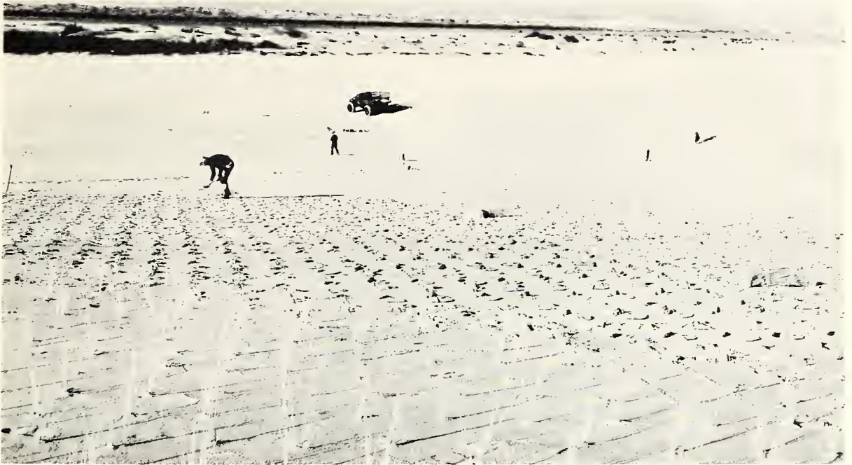
Photo 38.--Crew planting European beachgrass to help stabilize the shifting sands. SCS photo NO. 7-1529-2
